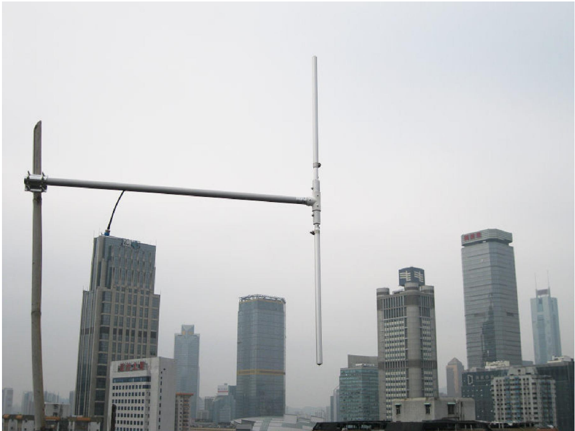
D. Finished Installation (We didn't connect the cable in this manual, in real operation, please connect the cable to the antenna after installation)
